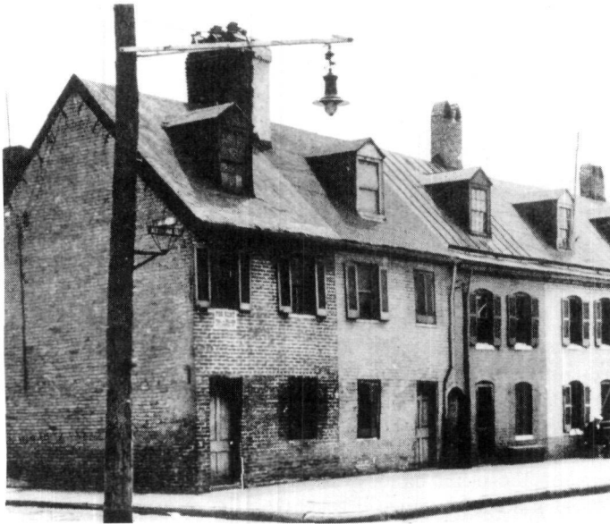
FIGURE 3. Baltimore row houses built about 1800. Source: R. Howland and E. Spencer, The architecture of Baltimore .
