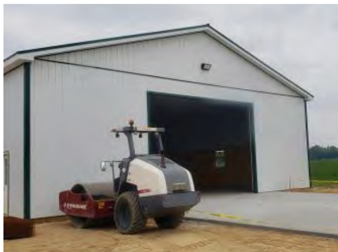
One of two new pole barns constructed for the wood products business and partially funded by the MARBIDCO WPIEI grant.
