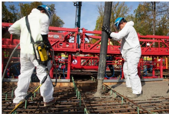
Crews pouring concrete on the bridge over Rock Creek.
