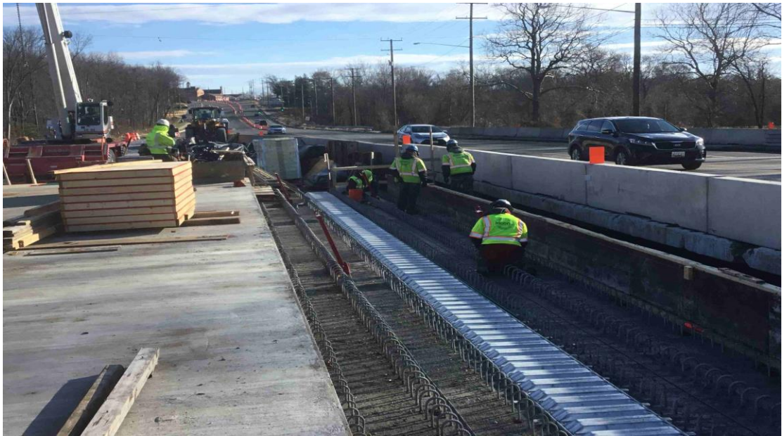
The Northwest Branch Bridge under reconstruction on University Boulevard in Adelphi
