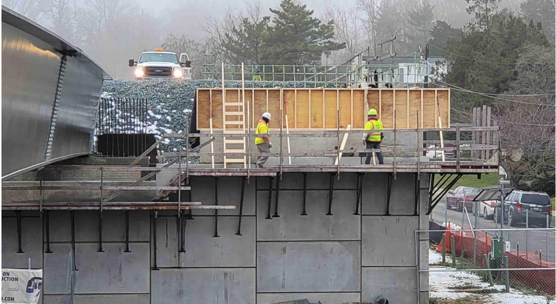
Formwork being finished at Connecticut Avenue in Chevy Chase Lakes
