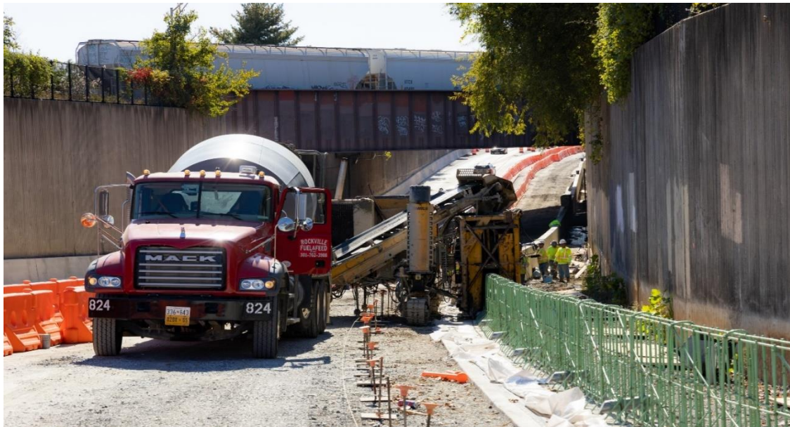
Retaining wall installation on Campus Drive in College Park
