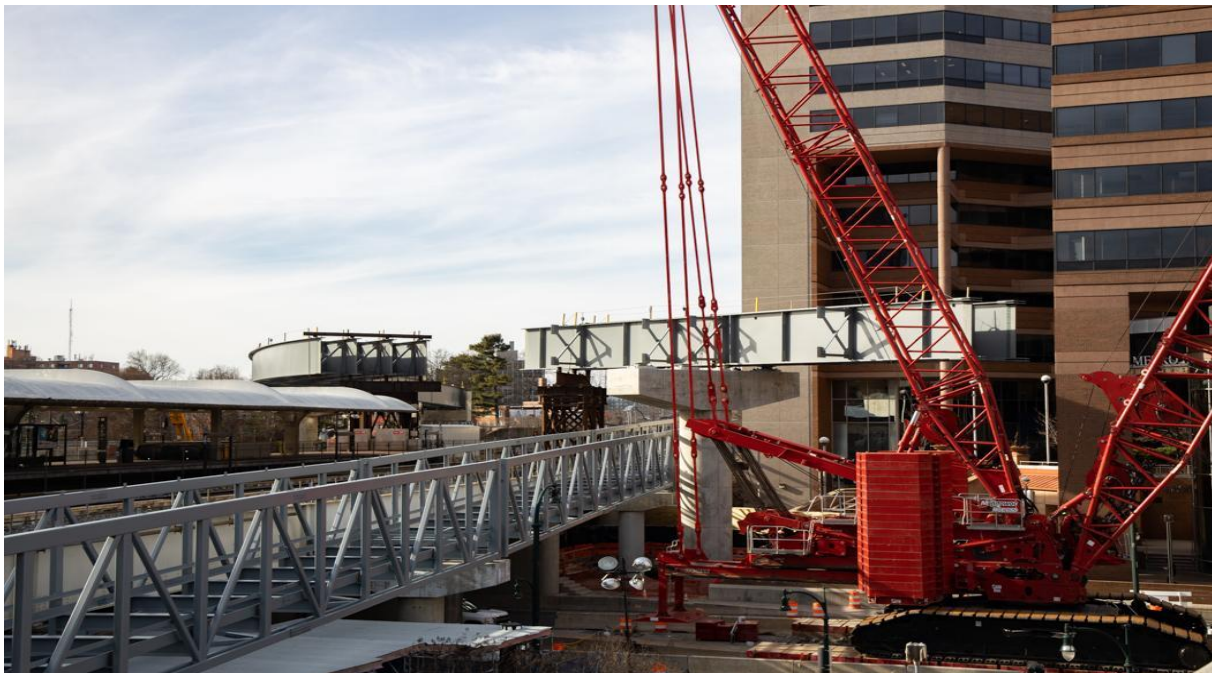
Girder Installation at the Paul S. Sarbanes Transit Center in Silver Spring
