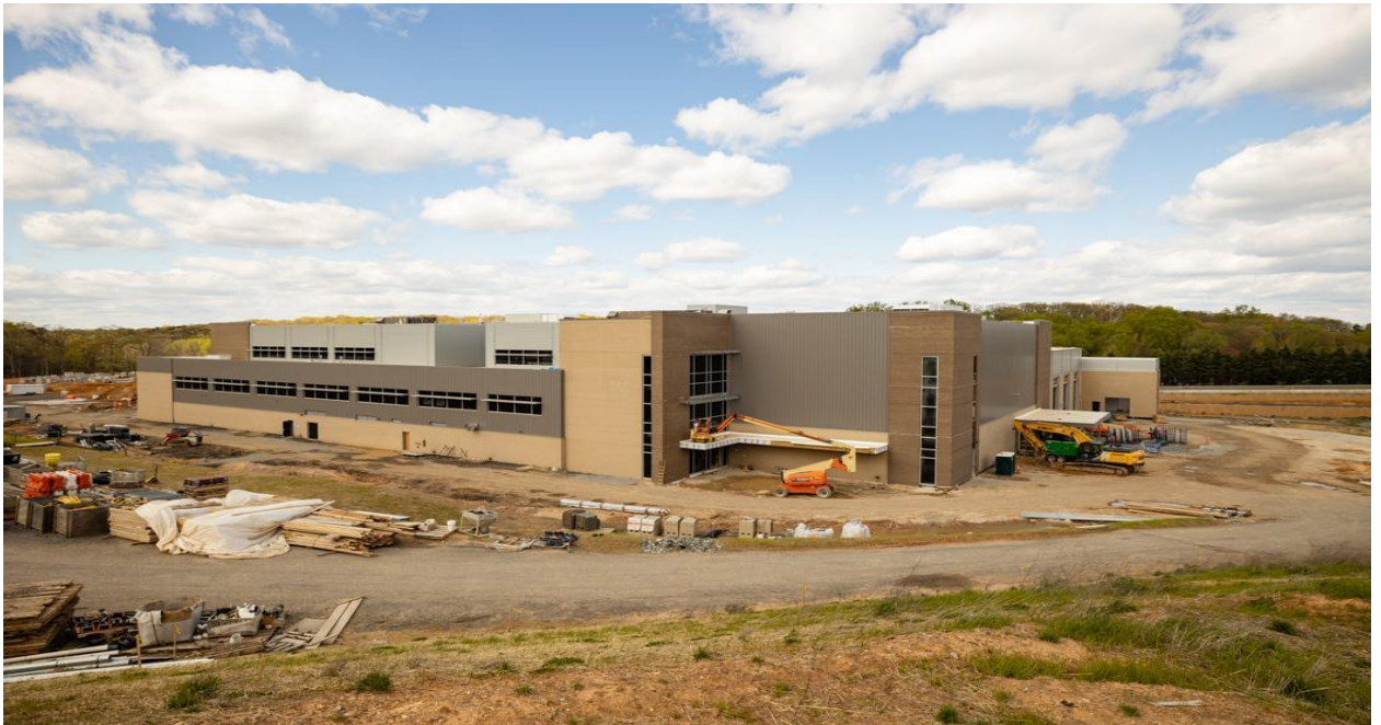
The Glenridge Operations and Maintenance Facility is near completion
