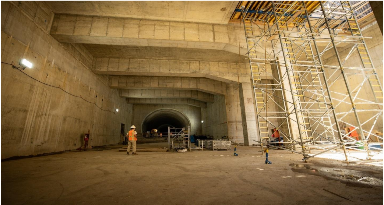
Final Touches Are Applied to the Manchester Place Station and Tunnel
