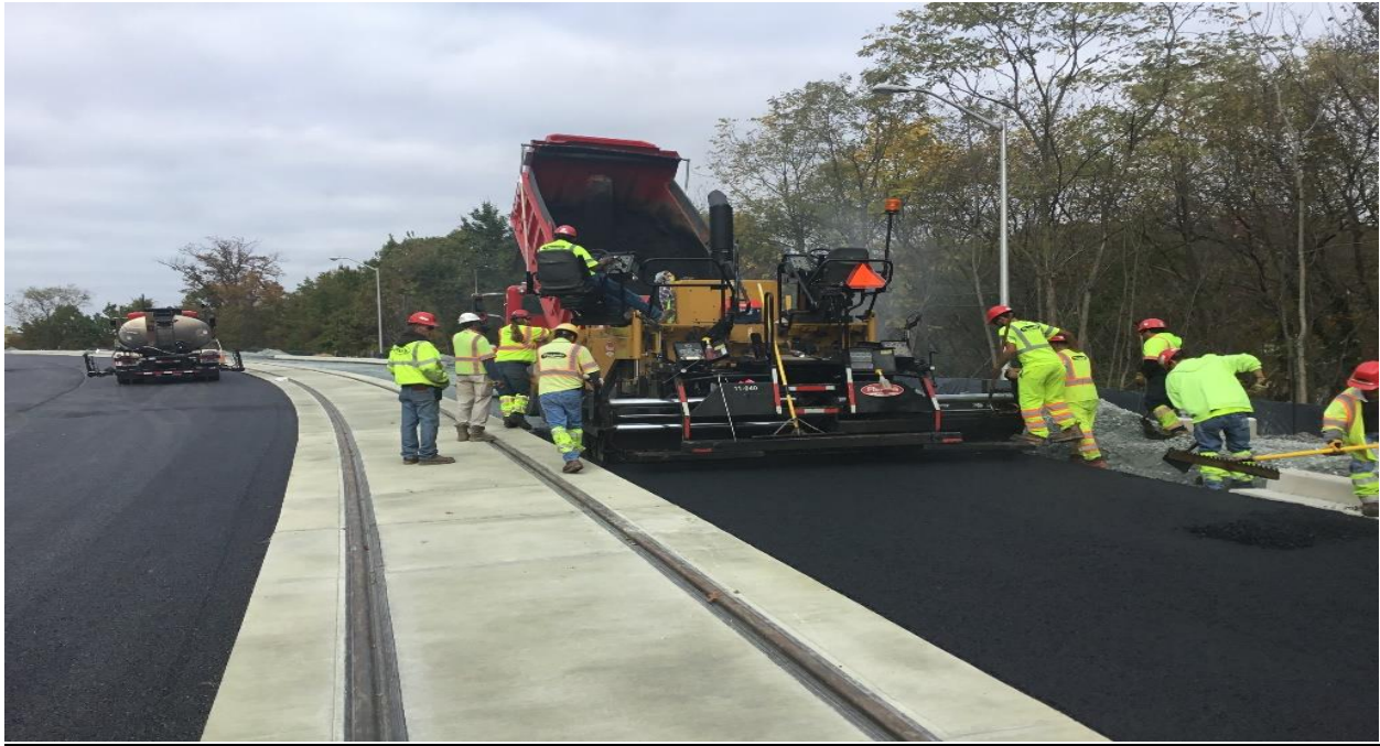
Asphalt Paving and Embedded Track at Ellin Road
