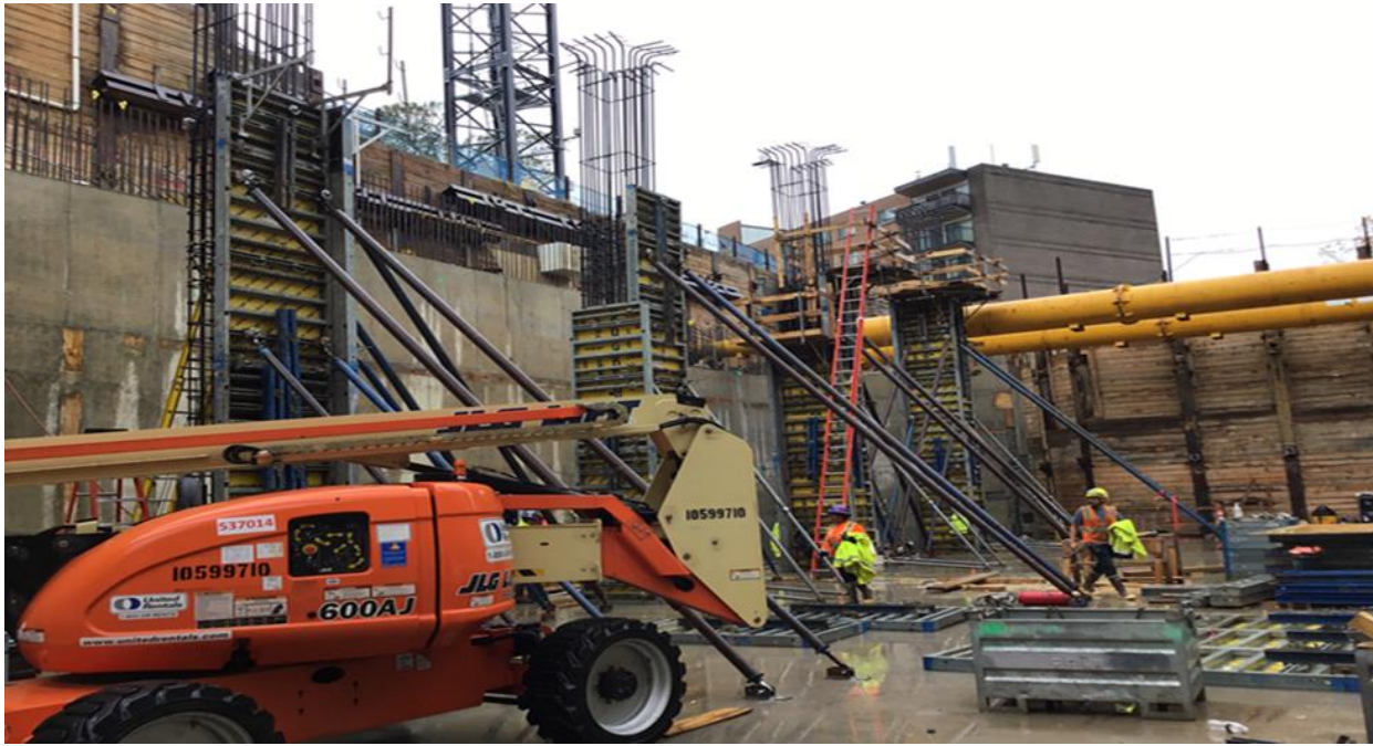
Concrete Formwork at Manchester Place Station
