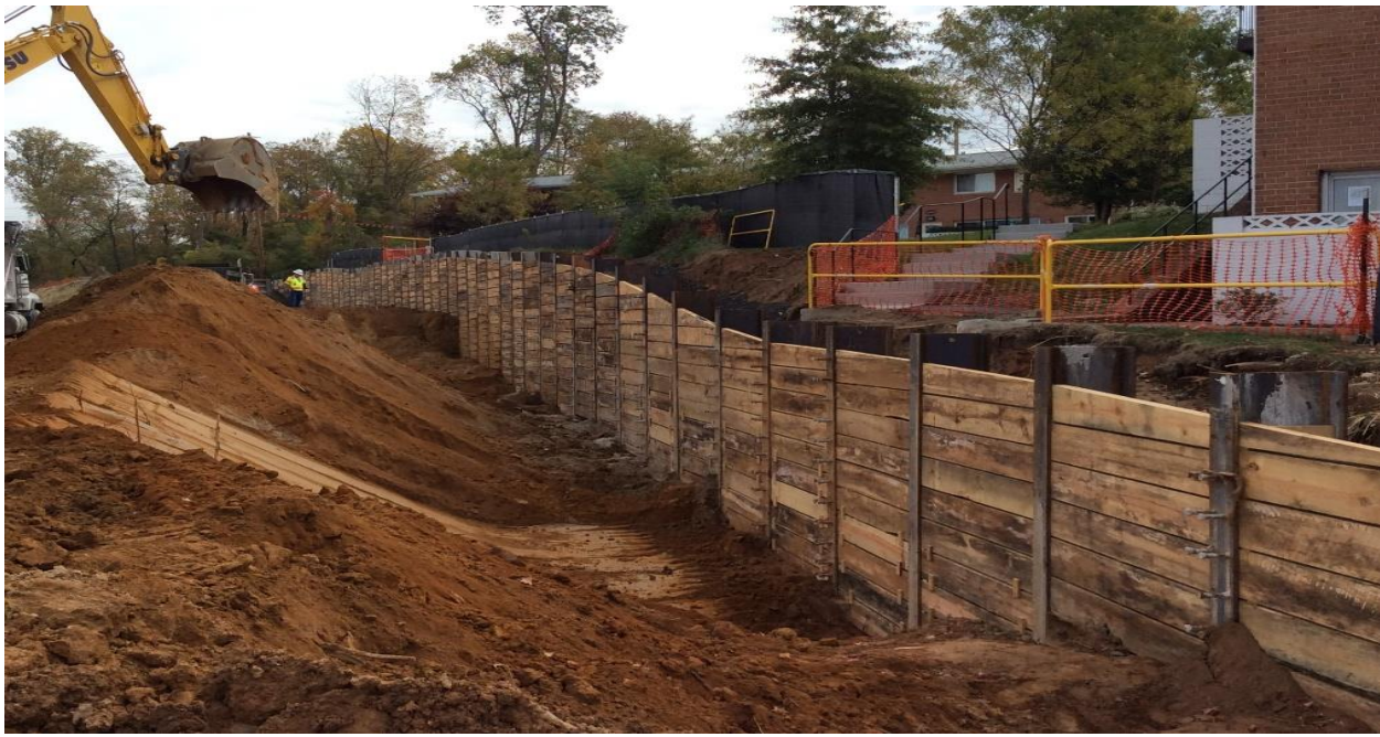
Excavation and Lagging for Retaining Wall 1-074 near Rock Creek
