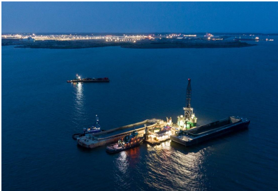
Dredging operations in the federal channels leading to the Port of Baltimore.
