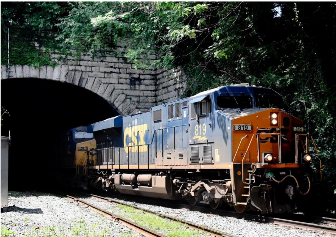
CSX Train Exiting the Howard Street Tunnel's North Portal
