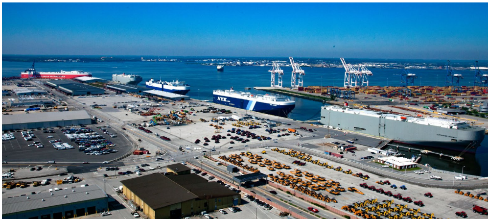
Busy day at Dundalk Marine Terminal
