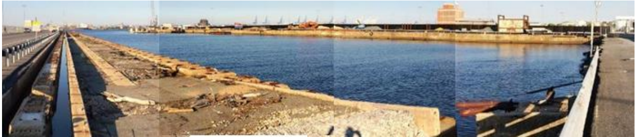
Fairfield Marine Terminal Wet Basin, September 2015.
