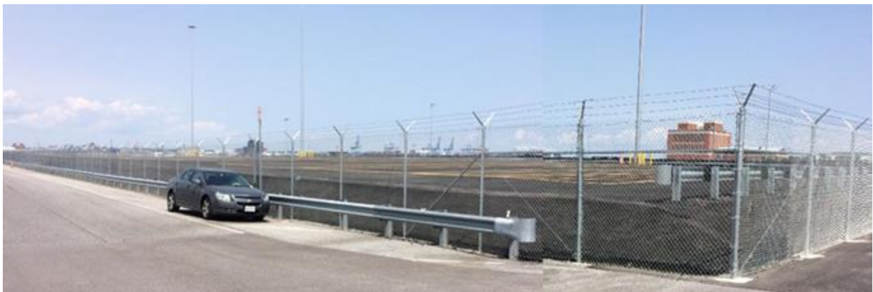
Fairfield Marine Terminal Wet Basin, Nearly Complete, July 2019.
