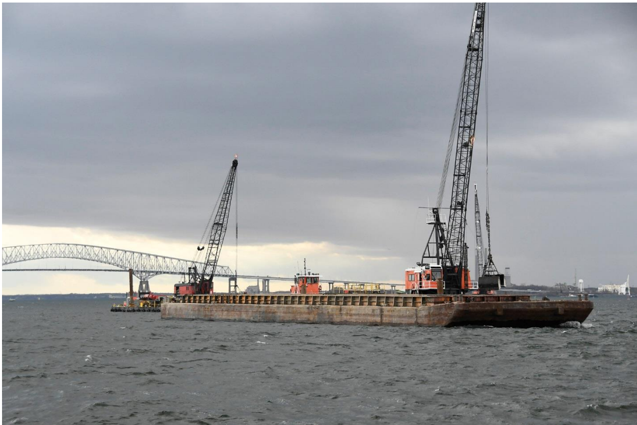
Dredging in the Baltimore Harbor Channel
