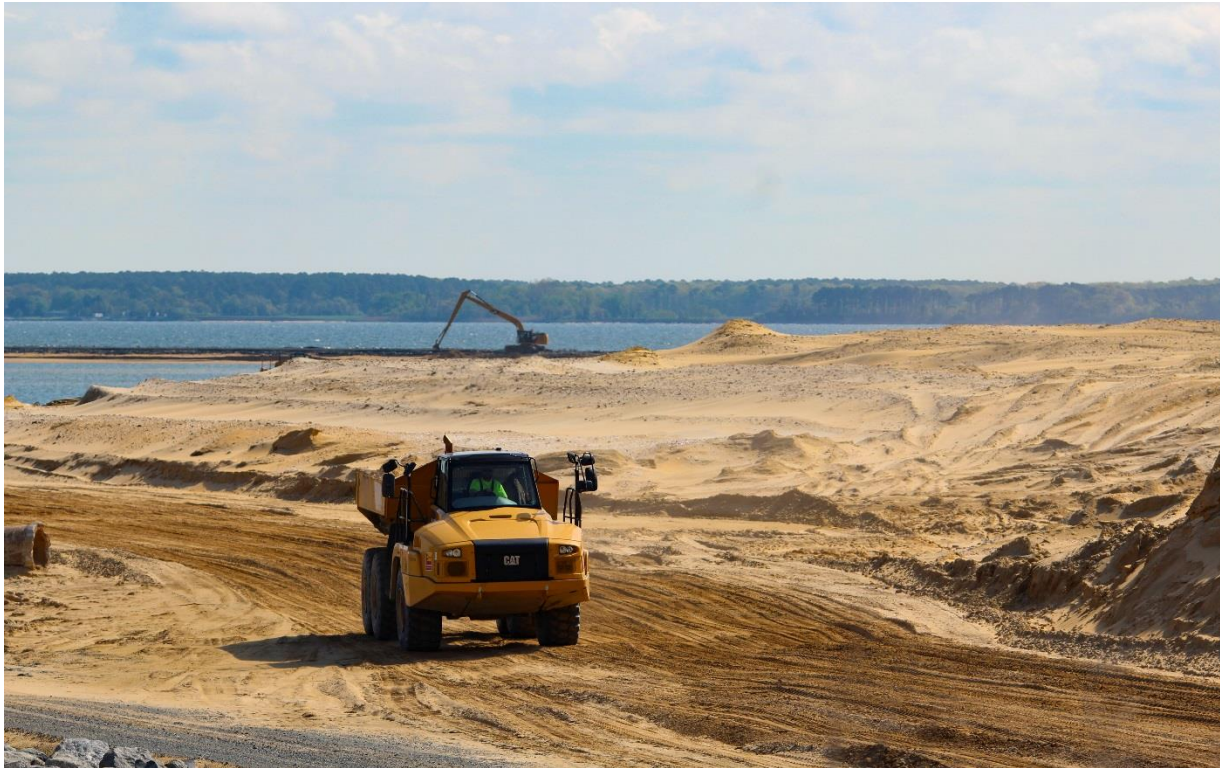
Expansion work underway at Poplar Island
