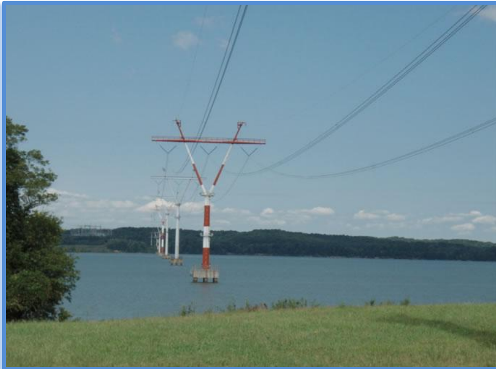
Figure 4-20 Existing 500-kV Transmission Line Crossing of the Potomac River
