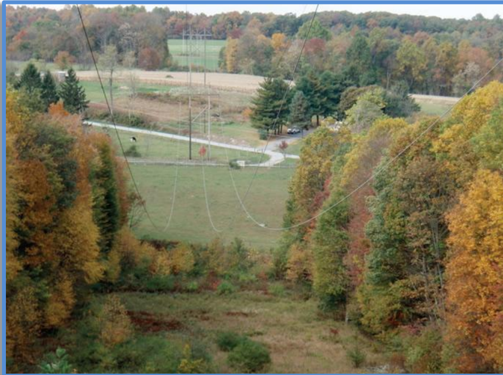
Figure 4-24 An Example of Typical Transmission Line Vegetation Management in Frederick County, Maryland
