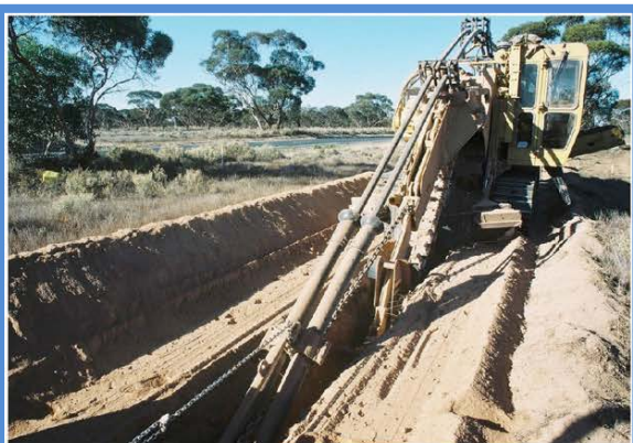
Figure 2-15 Direct-burial Underground Transmission Line Installation
