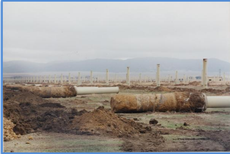
Figure 4-27 Decommissioning of the Carrizo Plains Power Plant
