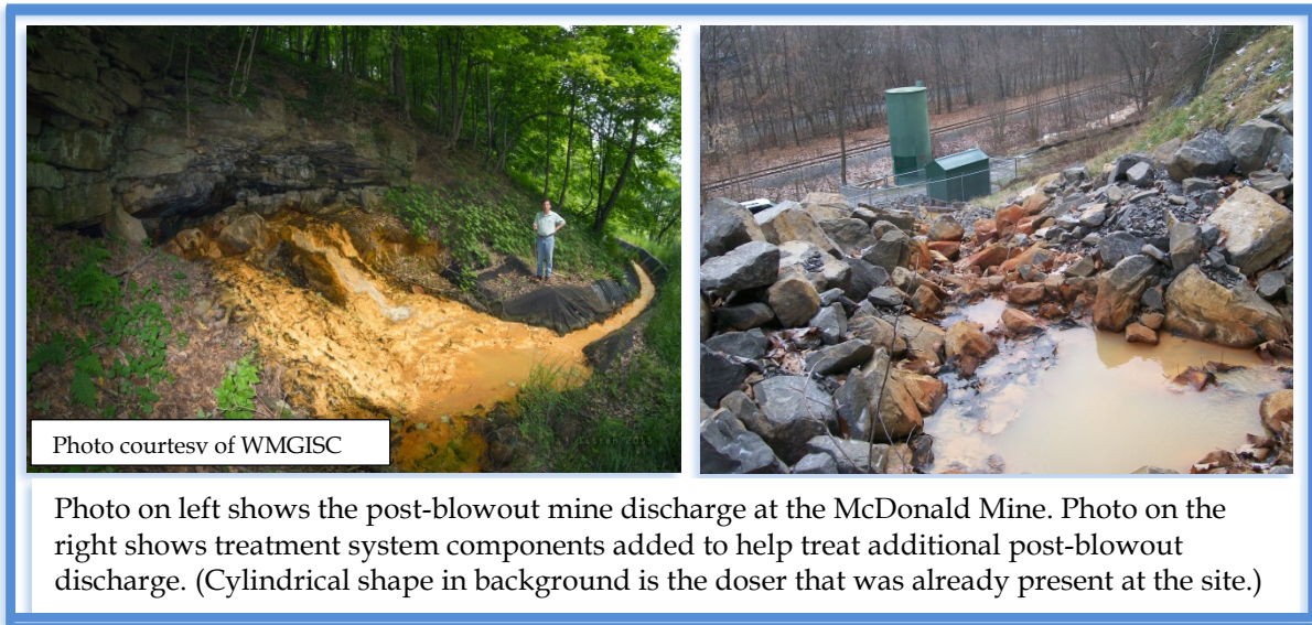
Figure 5-15 McDonald Mine Seep
