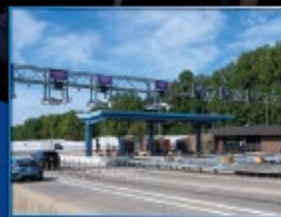
DULLES TOLL ROAD
