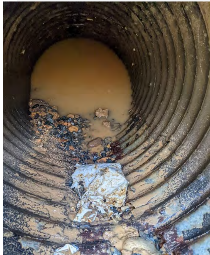
Above: Stormwater Structure Repair Right: Stormwater Inspection, BWI Airport
