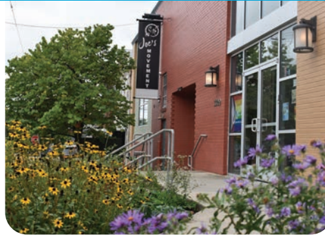
Joe's Movement Emporium installs a variety of practices on their campus: a green roof, rain gardens with native species, a mural, and a kinetic water sculpture.
