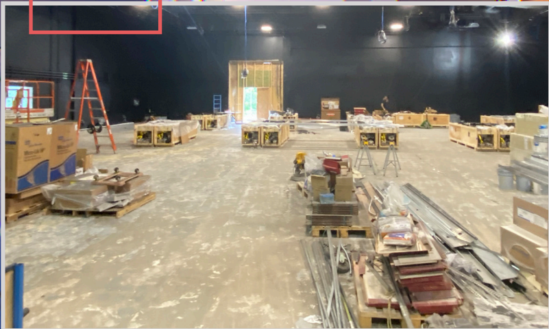
Inside of the Kaplan Studio during construction in June 2021.
