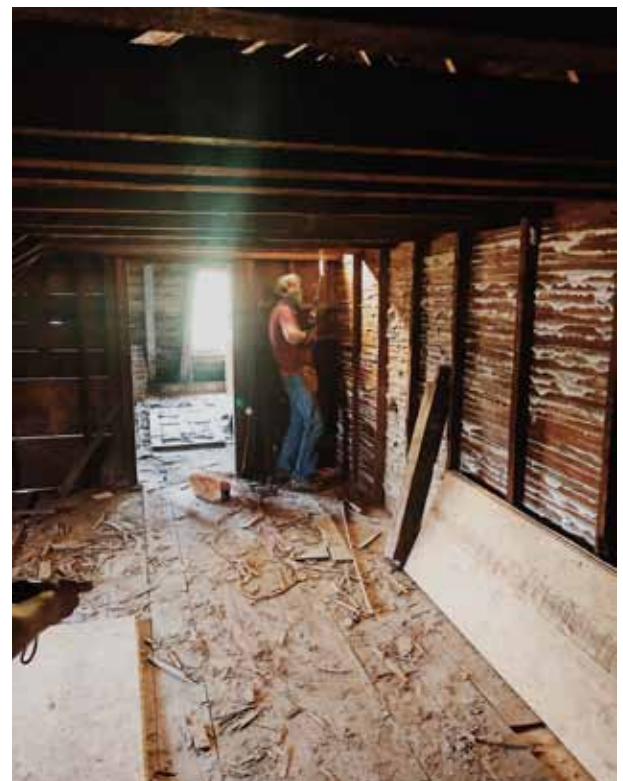
Dendrochronologist Mick Worthington takes core samples from the rafters of Appleby, a house in Cambridge. Analysis and comparison of tree ring data determined that Appleby was constructed with timbers felled during the summer of 1771.
