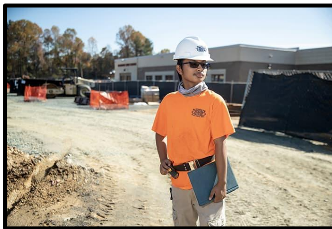
Christopher Borja, youth apprentice with Altimate Electric, Inc., at his worksite Hammond High School, a Howard County Public School System facility.
