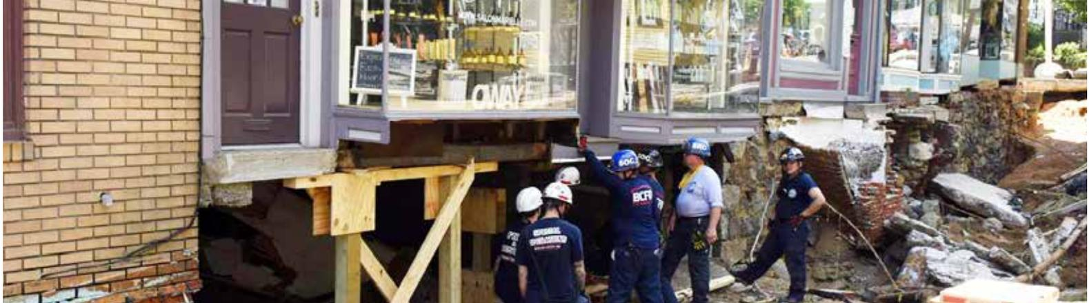
▲ Workers stabilize a building before digging could begin to repair a broken water main in Ellicott City after the historic flooding on July 30, 2016.
