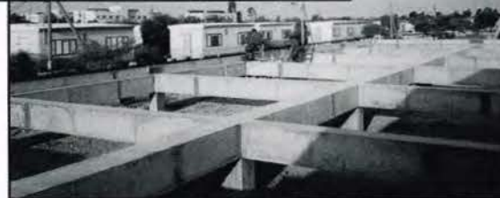
“Operation INCA 98”, construction of dormitories in Israel
