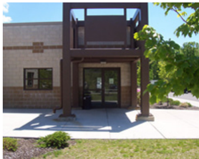
Mid-Atlantic Luzerne hardware secure facility located in PA
