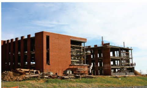
Construction of the Dundalk High School in Baltimore County.
