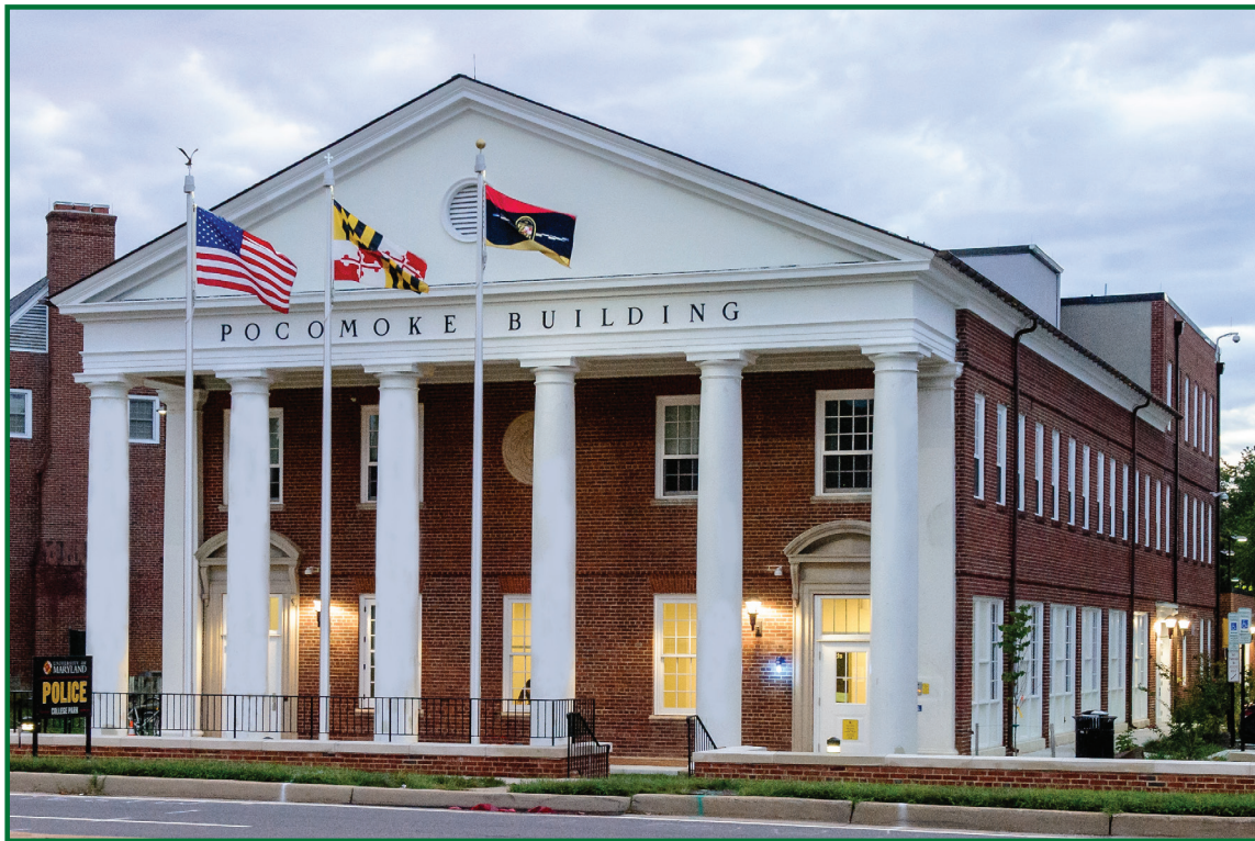
Pocomoke Building, University of Maryland College Park, Prince George's County
