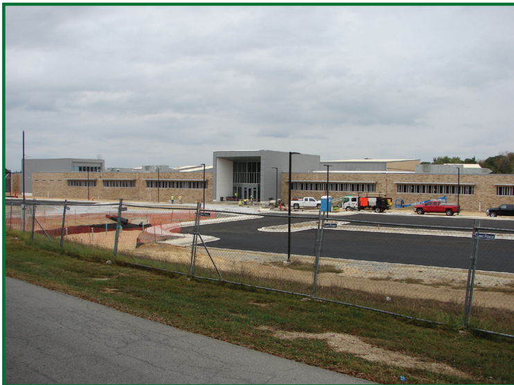
Cheltenham Youth Detention Center, Department of Juvenile Services, Prince George's County, construction photo
