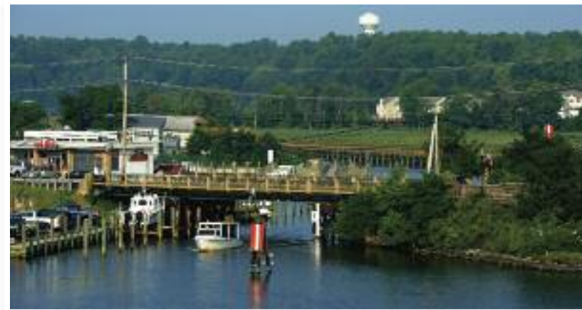
The project to replace Fishing Creek Bridge is scheduled to go to bid later this year.
