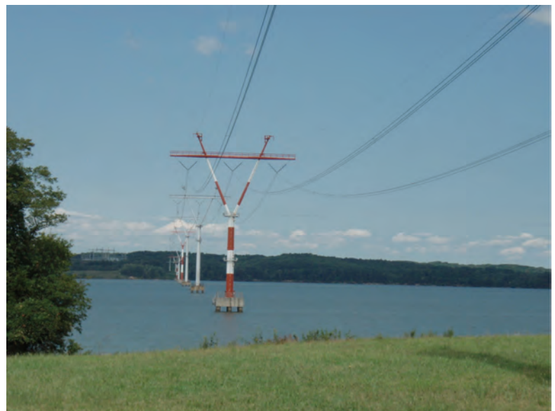
Figure 4-29 Existing 500-kV Transmission Line Crossing of the Potomac River
