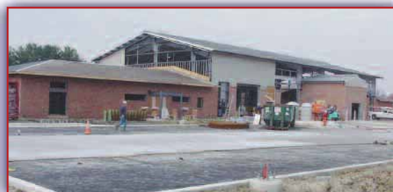
The Dundalk Field Maintenance Shop at 60% completion. When operational, by the summer of 2008, the shop will support Maryland Army National Guard units throughout the Baltimore area, increasing readiness for state and federal missions.
