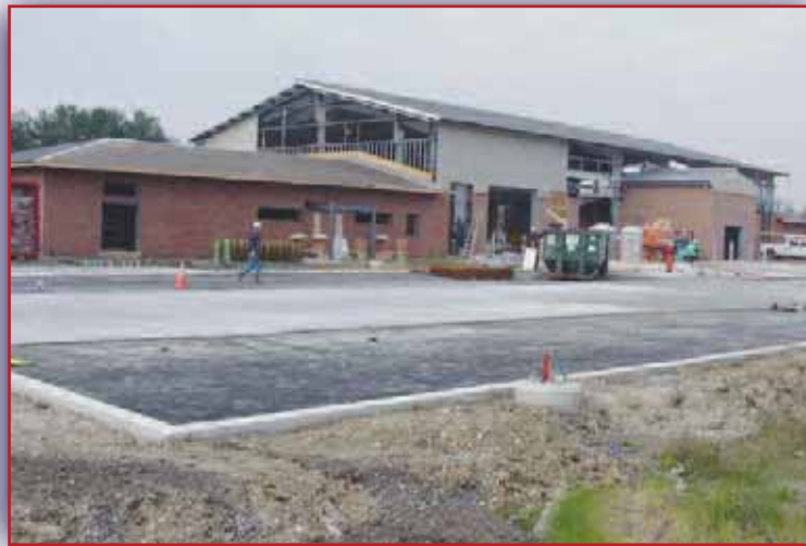
The Dundalk Field Maintenance Shop is at 60% completion. The shop will be operational by the summer of 2008.
