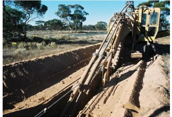
Figure 3-25 Modern Underground Transmission Line Installation
