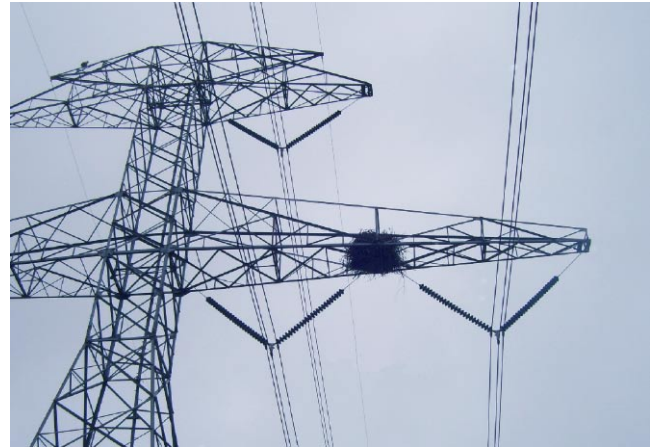
Figure 3-24 Photograph of Eagle's Nest in Tower
