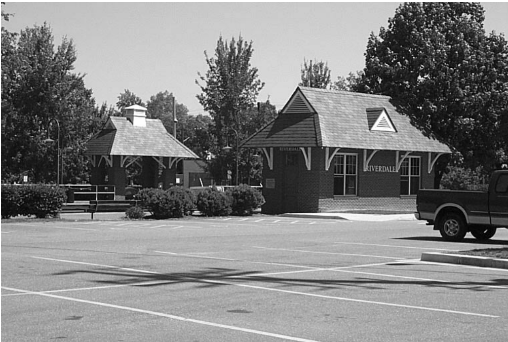
Riverdale Train Station
