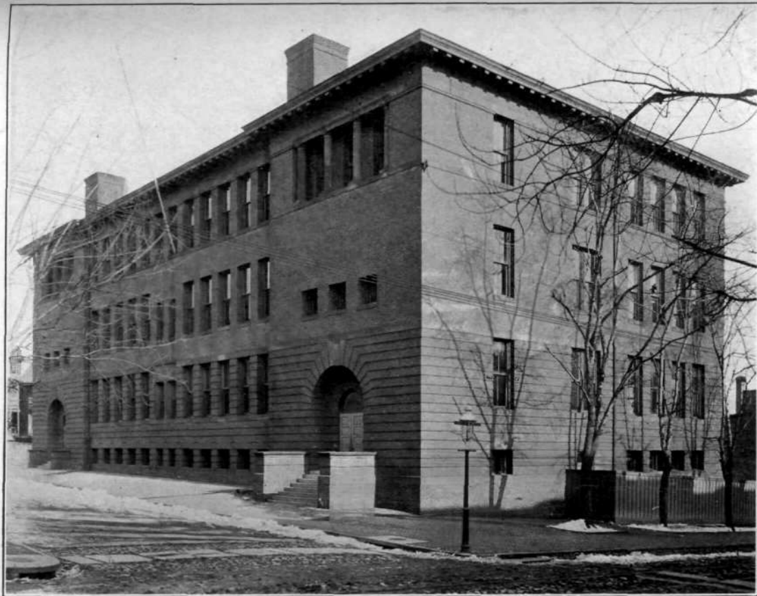
SCHOOL No. 61—LINDEN AVENUE AND KOENIG STREET
