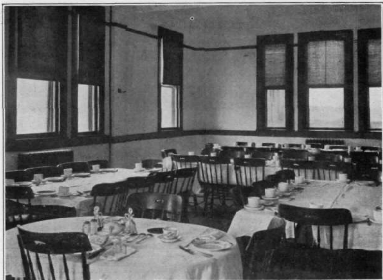
A COTTAGE DINING ROOM
