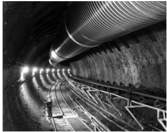
View of an exploratory tunnel dug by the 25-foot diameter tunnel boring machine at Yucca Mountain. Photo courtesy of the U.S. Department of Energy.
