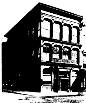
The cast-iron elegance on Baltimore Street before the fire of 1904 was copied on a less grand scale elsewhere in the city. The Oldtown site still stands today.
