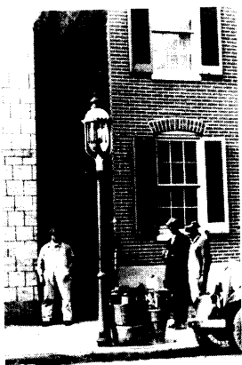
Little Rock Street, which extended from Lexington Street to Saratoga Street, was one block long and only six feet wide for one-third of its length, yet the street contained thirty-five houses and a stable.
