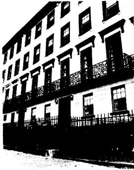
A once grand residential row, Waverly Terrace was rehabilitated in the 1970s by the city of Baltimore for use as apartments.
