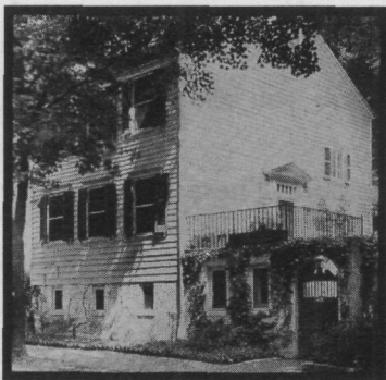
Volta Place after remodeling
