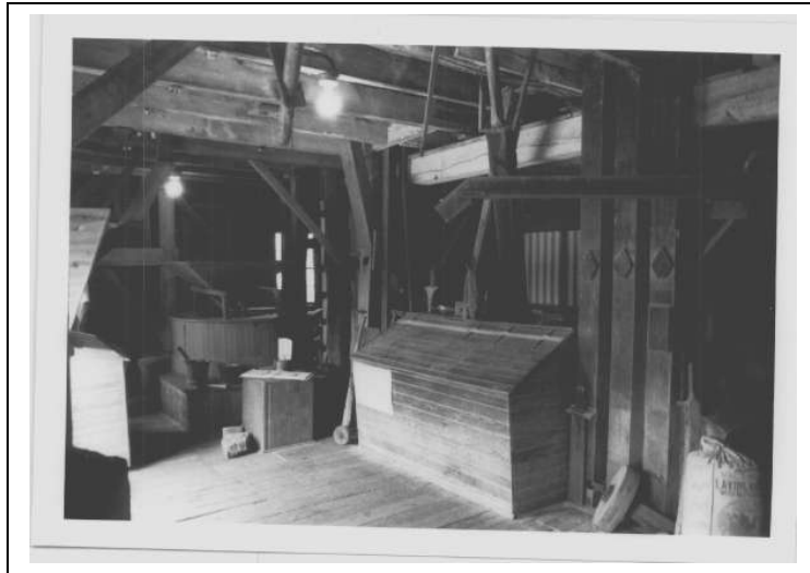
Wye Mill, elevator conduits, MHT photo by Nancy Miller Schamu.
