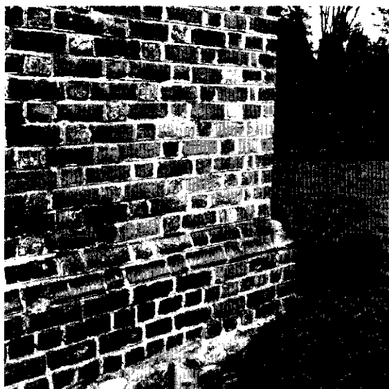
The outer walls of Smallwood's restored house are laid in Flemish bond, while the watertable is executed in English bond. This combination of brick bonds was popular in Southern Maryland colonial architecture.
