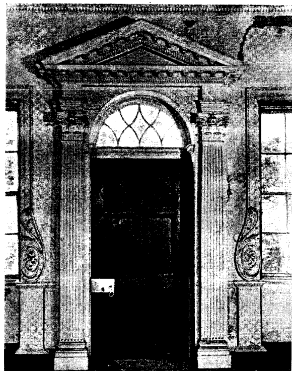
Door and Window Trim of the Great Hall; Probably from Buckland's Workshop
