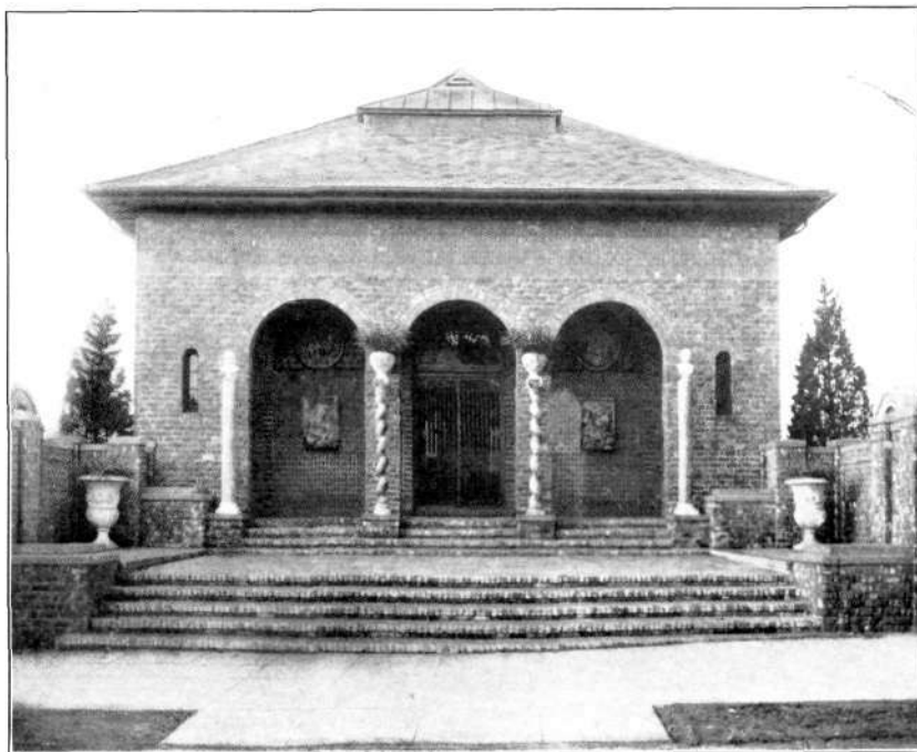
Museum. Main Entrance. Addition of 1913.
