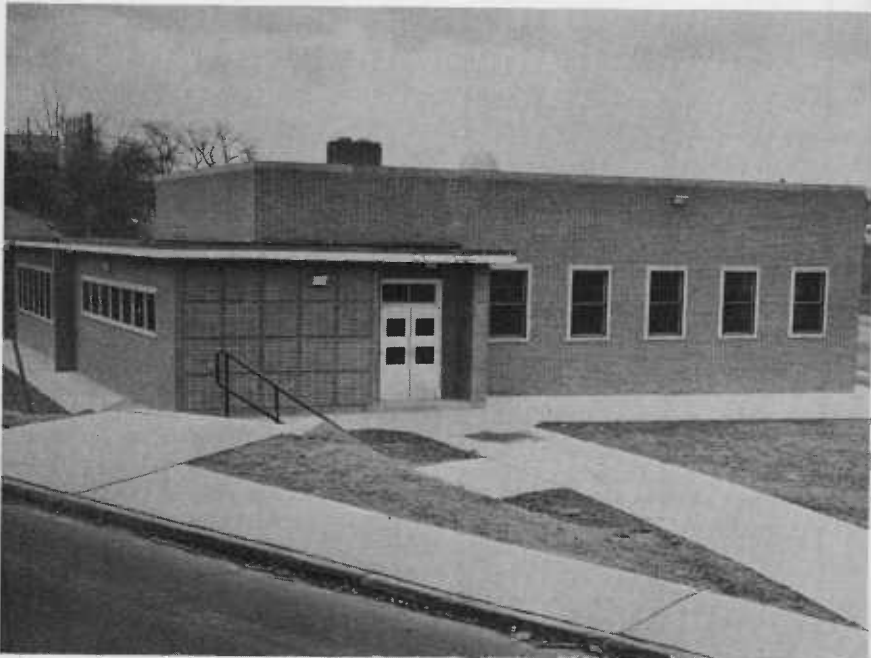
Gwynns Falls Recreation Center Completed in 1962
