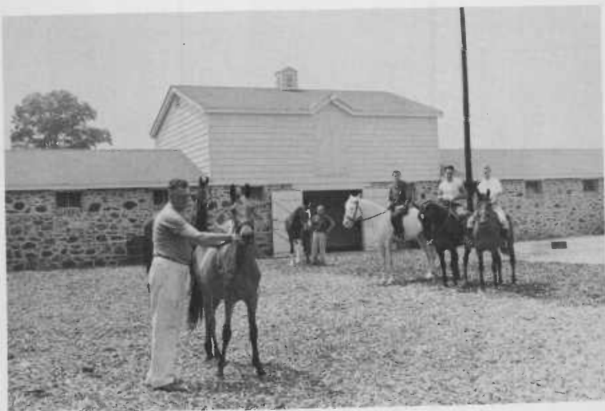
New riding academy and stable—Leakin Park.
